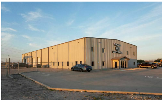
3174 CR 48, Robstown, TX 78380 Net Leased Heavy Industrial Facility | Sale: $5,000,000 For more information, contact John Foret john@craveyrealstate.com | 361.271.1527
